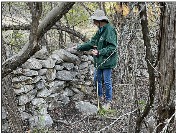
Fig. 2. Part of wall showing its original 3-foot height. Photo by Mackenzie Brown
