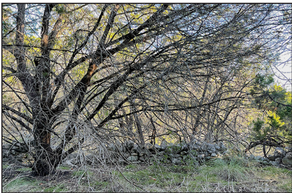
Fig. 1. Old, crumbling “German” wall on Honey Creek trail. Photo by Mackenzie Brown
